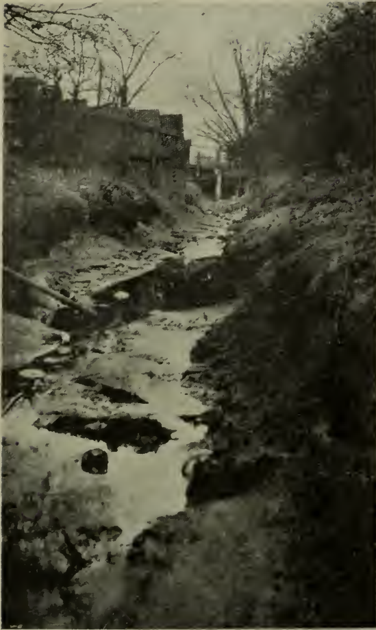
FIG. 29. DUKE'S DITCH, CHISWICK. (Before construction of Culvert.)
